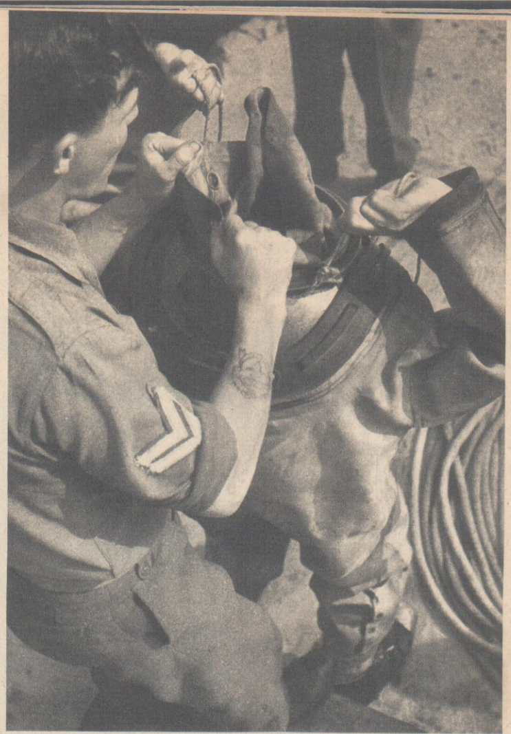
Below: Divers' bootlaces are made of thick tarred rope. The boots, capped with brass, weigh 19 pounds each.
