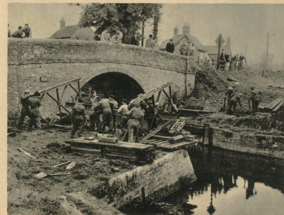
The canal bridge has been “blown.” Sappers build a Bailey to carry Southland Centurions.
