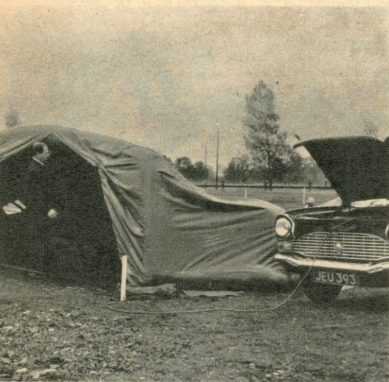
Above: This inflatable hut can be blown up in two minutes by a motor-car battery and packed into a car boot. Below: The cargon freighting system demonstrated by two soldiers pushing a loaded container on to a waiting lorry.
