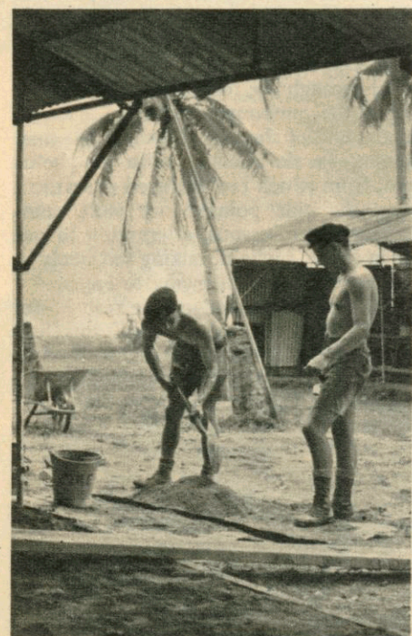
Above: A massive tractor-towed scraper levels the approach road to the rifle range firing point. Below: Mixing concrete for the floor of a NAAFI store in camp. Cement was not easily come by, but sand was plentiful!
