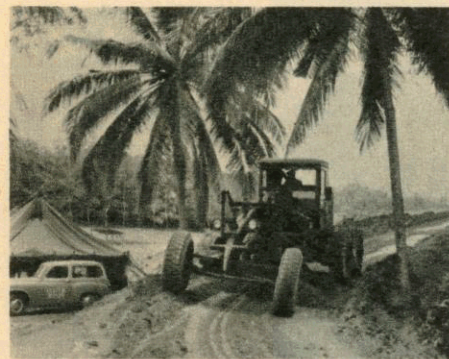
A Blaw-Knox grader puts the finishing touches to a new road leading down to the Sappers' tented camp on the beach.
