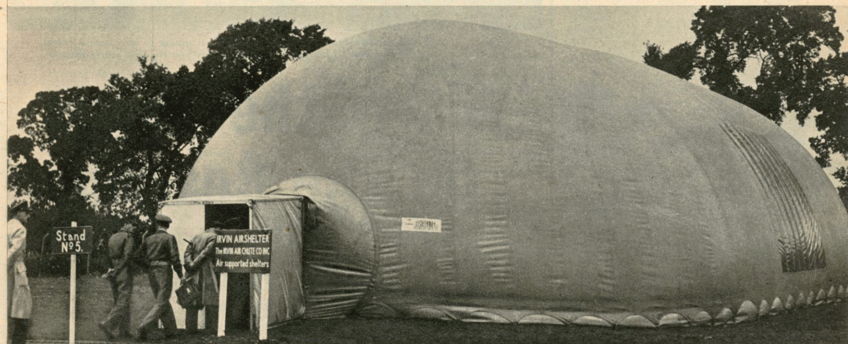
Above: The Irvin air shelter which has 40,000 cubic feet of storage space. It takes an hour to inflate.
