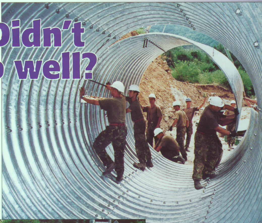
Full circle: Sappers bolt together sections of the pipe
