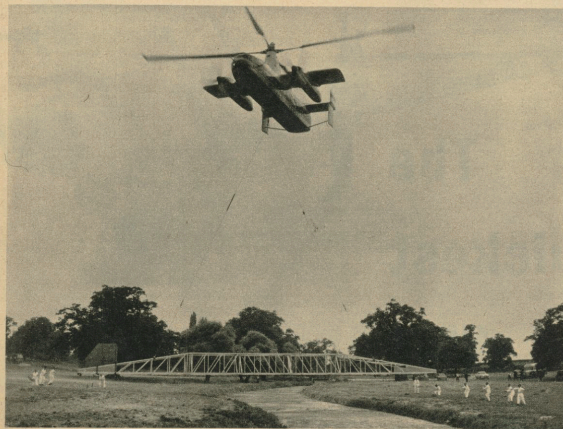
Hovering over the river in a park near Maidenhead, the "flying crane" slowly and accurately lowers the bridge.
