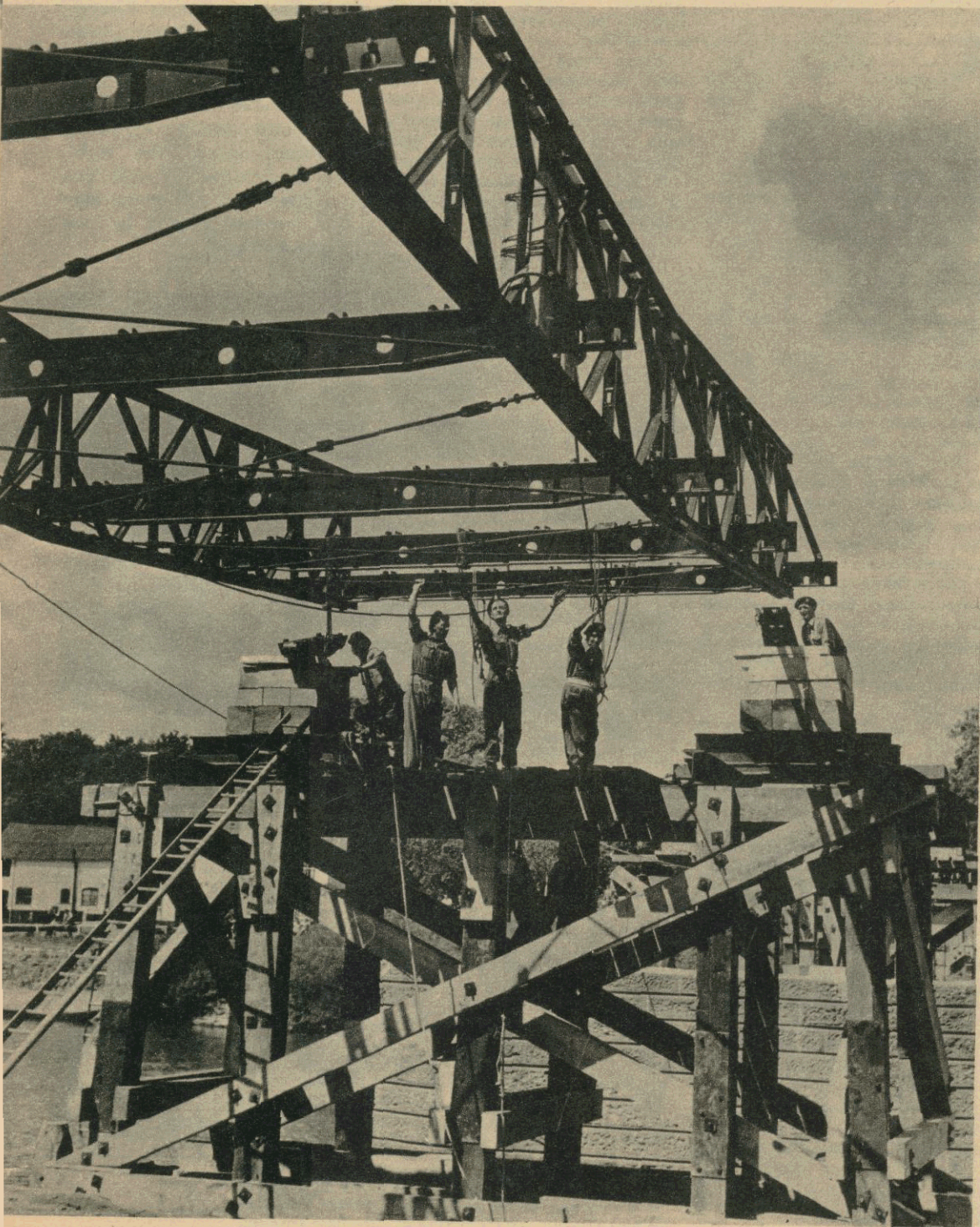
Men of the Royal Monmouthshires hoist into position a section of the 290-ft Bailey Bridge which they erected in three days over the River Haw near Gloucester. When the old bridge was wrecked by a barge, traffic made a 14-mile detour to cross the river.
